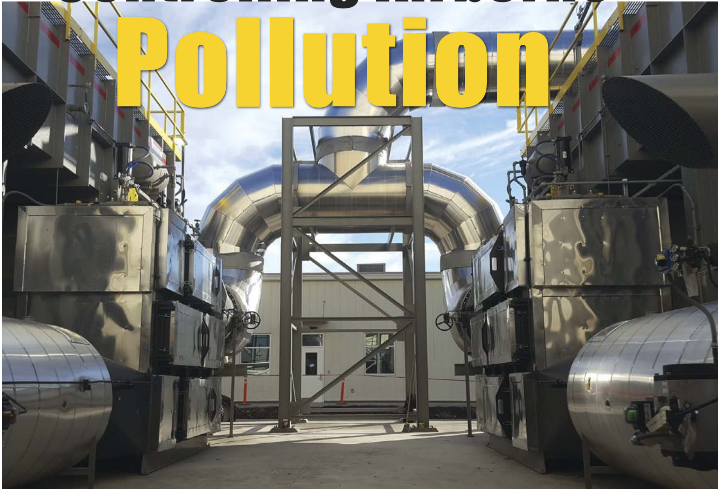
Two side-by-side Anguil model 200 Regenerative Thermal Oxidizers installed at a California facility.
